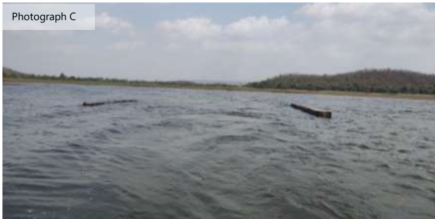
Photograph C: South-eastern part of Dev (Deo) Reservoir [Tadiya Lake] (354004 mE, 2474016 mN) with shallow water depth and submerged construction work.
