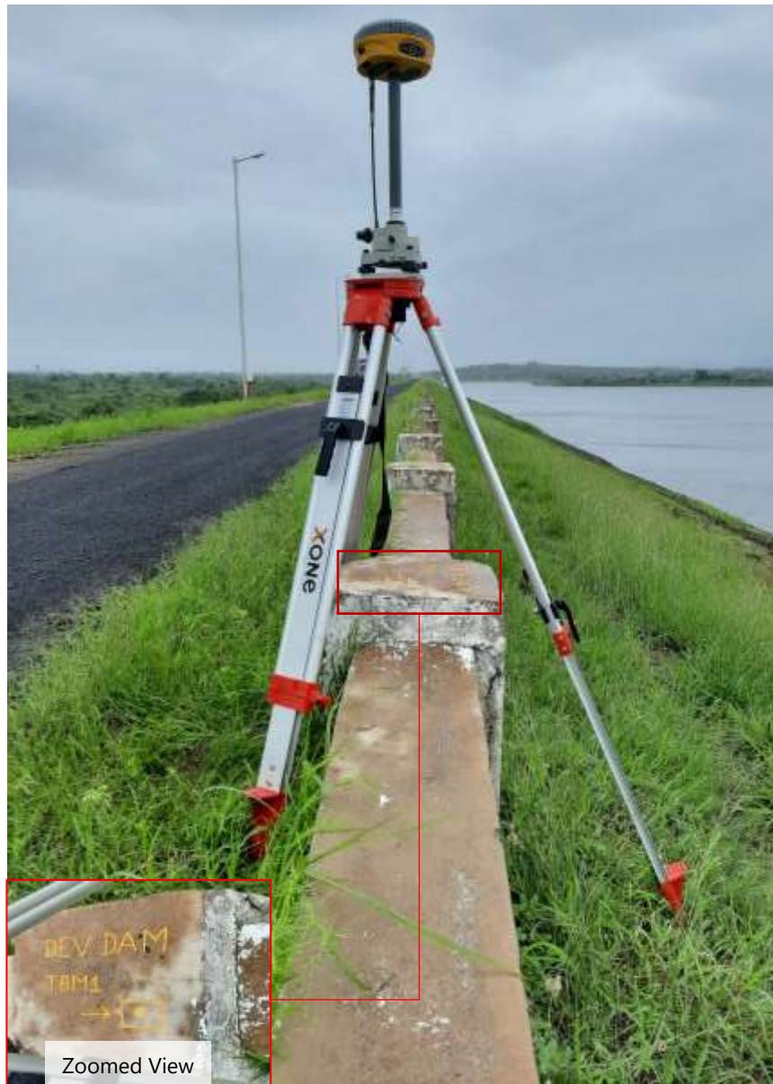
Figure 3.1: Temporary Benchmark 1 (TBM1)
